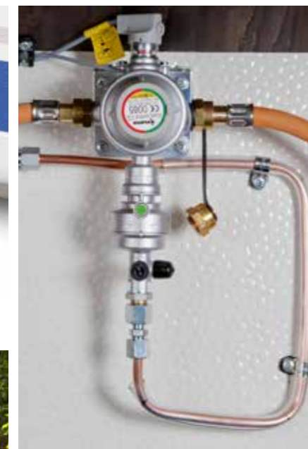
A gas changeover regulator automatically switches to the reserve bottle when the first is depleted.
